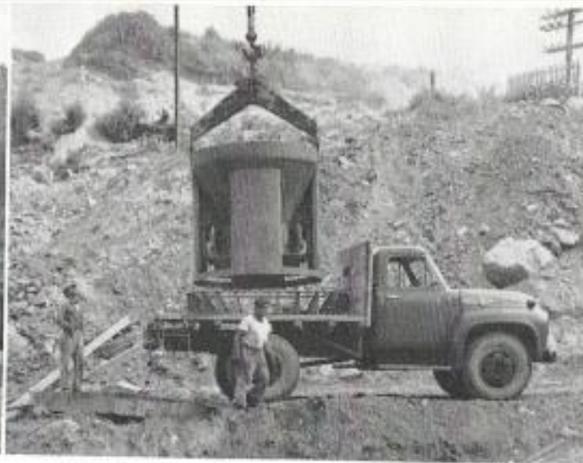
By the dam site crane lifts bucket from truck to the monolith under construction.
