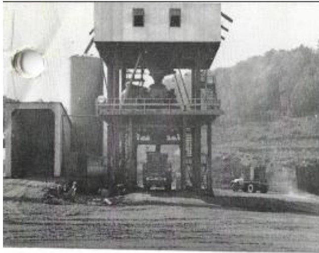
From bin below mixing plant fresh concrete pours into large bucket on truck.
